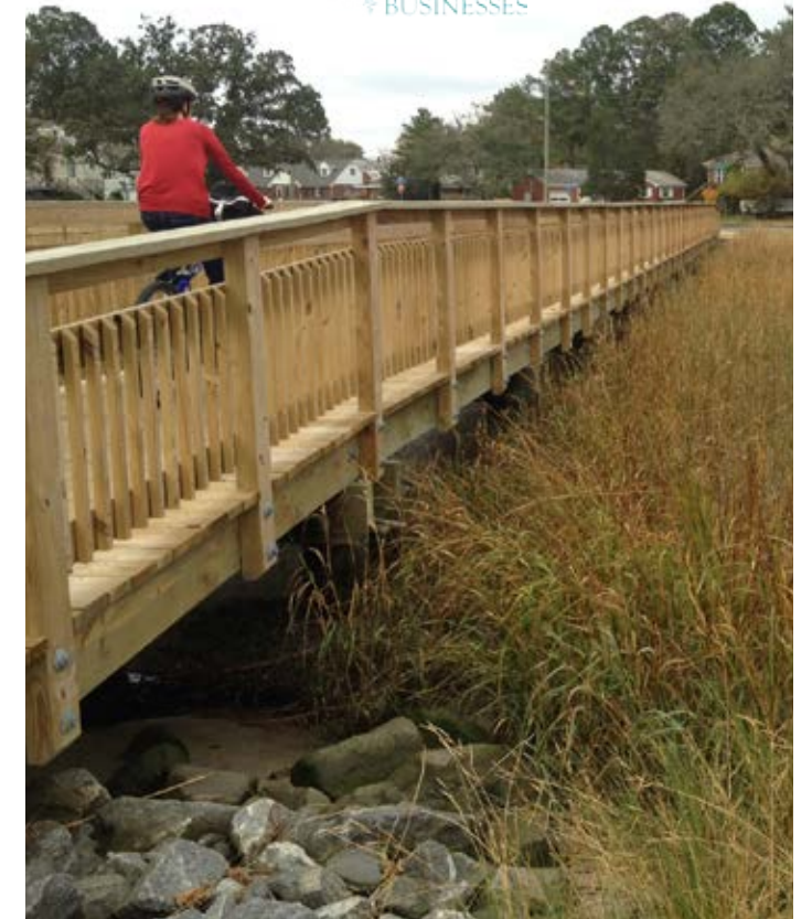
Norfolk's Environmental Stormwater Management Division earned Model Level River Star in 2015 for projects like this 15,500 sq. ft. marsh at Myrtle Park.
