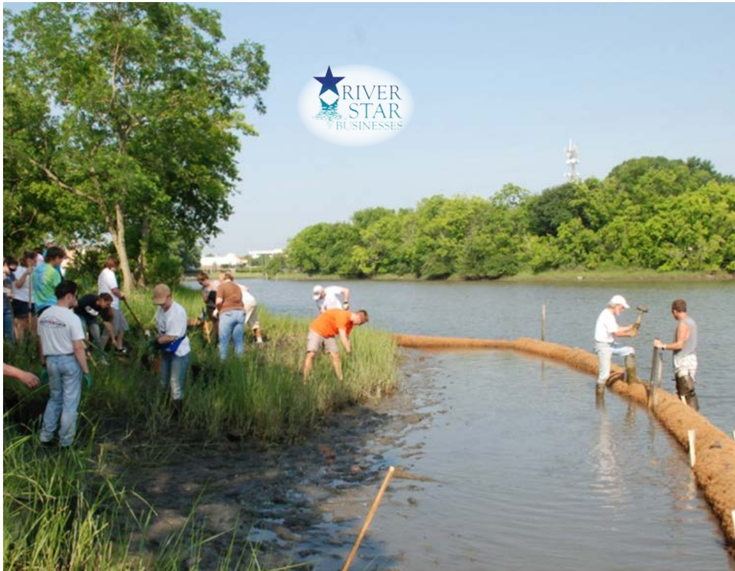
Lafayette Wetlands Partnership, other partners and volunteers establish a “living shoreline” on Colley Bay, part of the Lafayette branch. A “coir log” made of coconut fiber will protect the new wetland plants and stabilize the shore.
