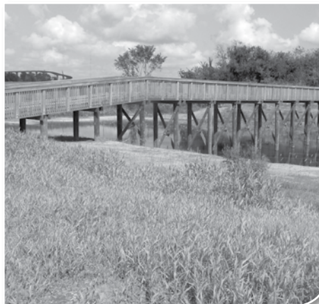
Businessman Bill Magann spearheaded construction of the pedestrian footbridge.
