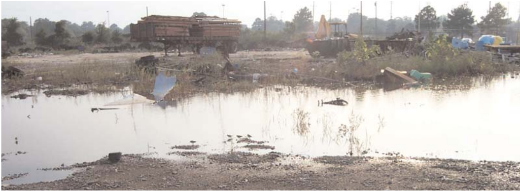
Runoff is a significant problem at the Peck site. Construction of a stormwater wetland is funded for 2002-03.
