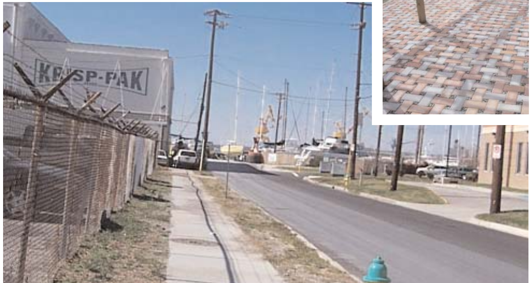
Southampton Avenue is discolored by parking lot sedimentation and runoff. This sidewalk can be replaced with permeable pavement (sample shown in inset), with a buffer along the fence.
