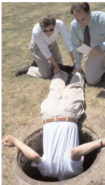
Investigators determined pipe slopes this way.
