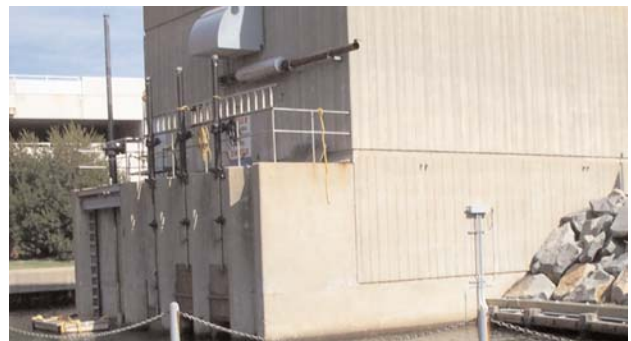
This lift station handles stormwater from 70 acres of downtown
