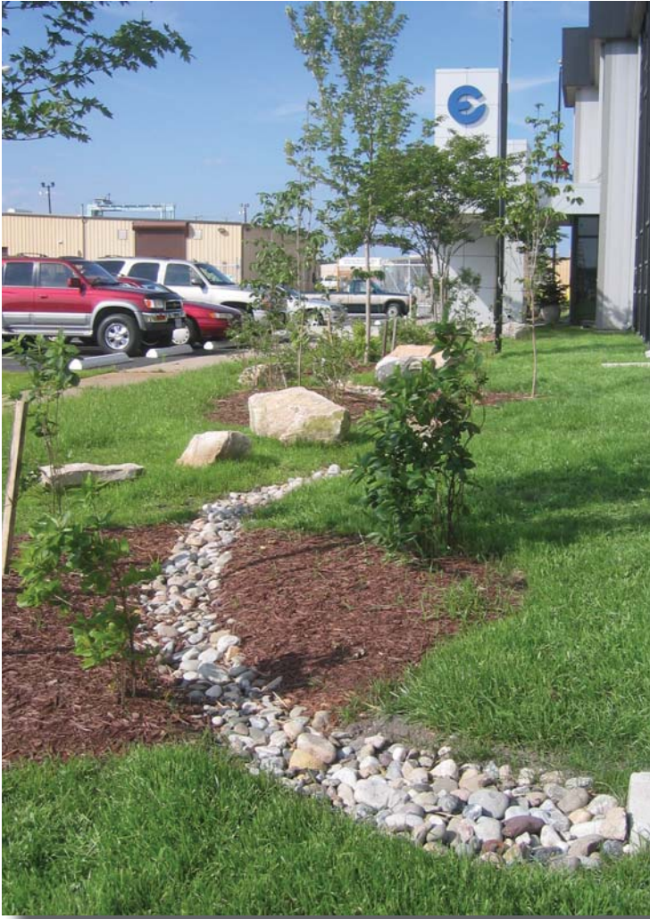
One of Earl's first projects was this rain garden or bioretention area that is landscaping that filters and reduces stormwater runoff at the shipyard's headquarters.
