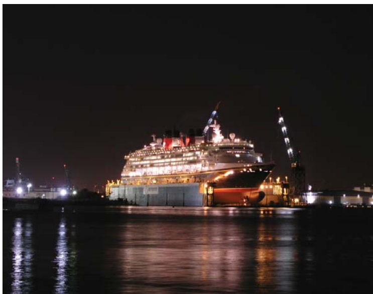
BAE Systems Norfolk Ship Repair (shown above) along with Norfolk Naval Shipyard treat the stormwater runoff as well as washwater from drydocks. Photo by Van White.
