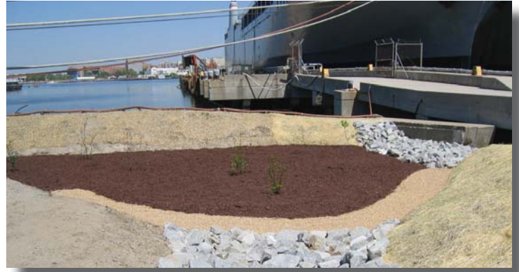
Retrofit in progress at Earl Industries.
