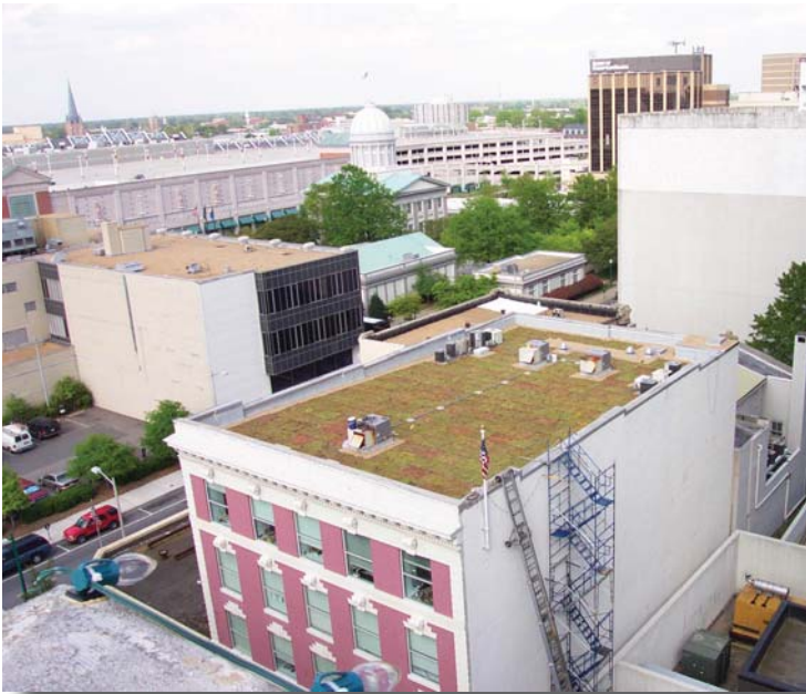
Atlantic Associates installed a green roof on its office building in downtown Norfolk.
