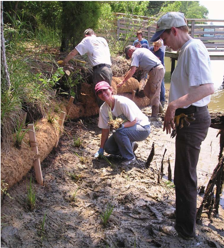
Volunteers install coconut fiber logs along a shore at Hoffler Creek Wildlife Foundation to reduce erosion. The logs were planted with wetland grasses for added habitat value as well as providing added erosion protection.
