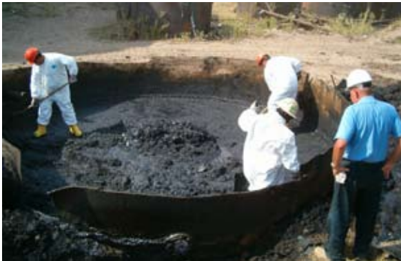
By 2006, the cleanup was underway. Here workers for the US EPA remove creosote in old tanks, reducing the potential for recontaminating cleanup areas in the river bottom.
