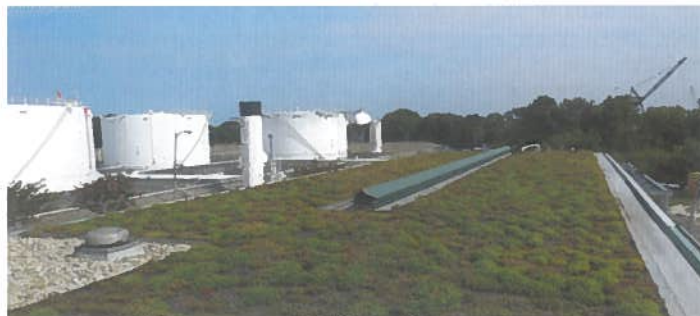
The green roof installation at the CITGO Chesapeake Terminal in April 2011 is planted with sedum. Right: Planted with slow-growing sedum, the green roof achieved full growth capacity by 2014. Photo by CITGO
