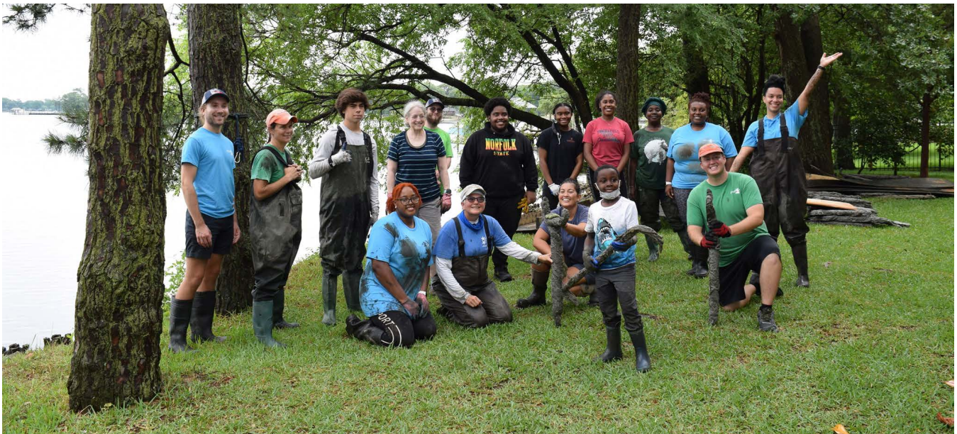
Norfolk State University students and community volunteers help construct an oyster reef using new innovative materials on the Eastern Branch. Photo by Elizabeth River Project/Joe Rieger
