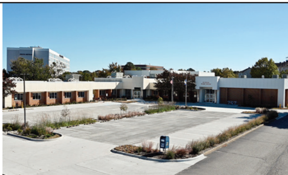
Hampton Roads Planning District Commission's (HRPDC) newly transformed parking lot captures 33,000 gallons of stormwater runoff and features recycled tire parking stops and native plants. Courtesy of HRPDC.
